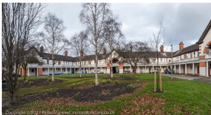
The former shopping centre in the Garden Village
