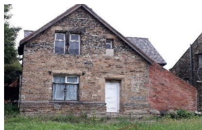
July 2020 : before renovation
