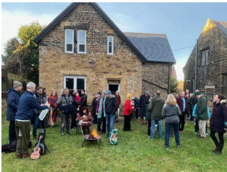
December 2023 Completion of Phase 1
